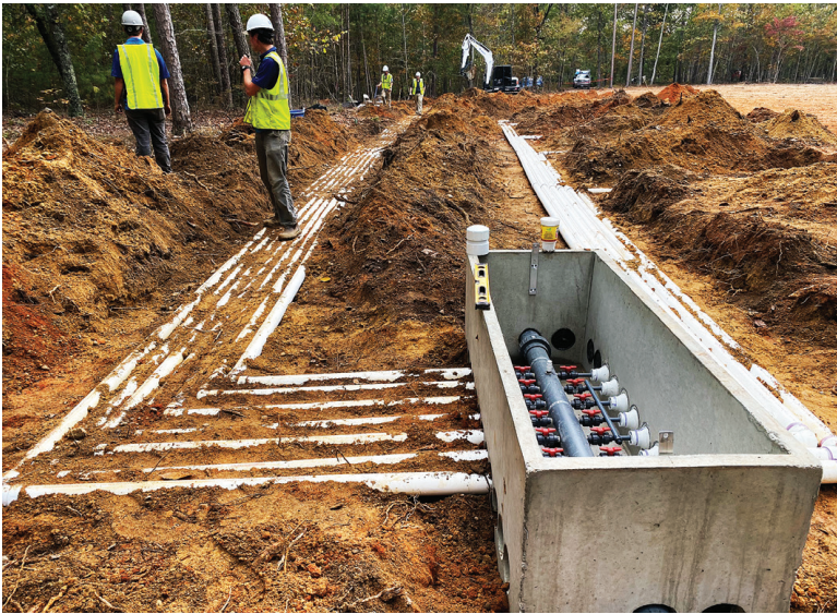
▲ A 14-tap manifold with supply lines.
